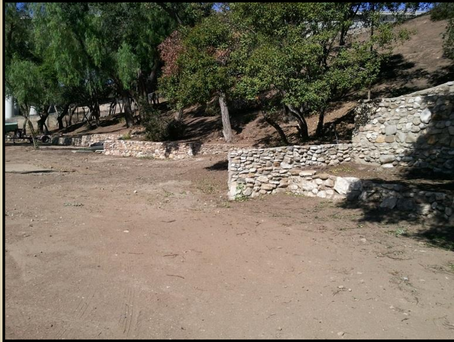
Retaining walls north of patio area
