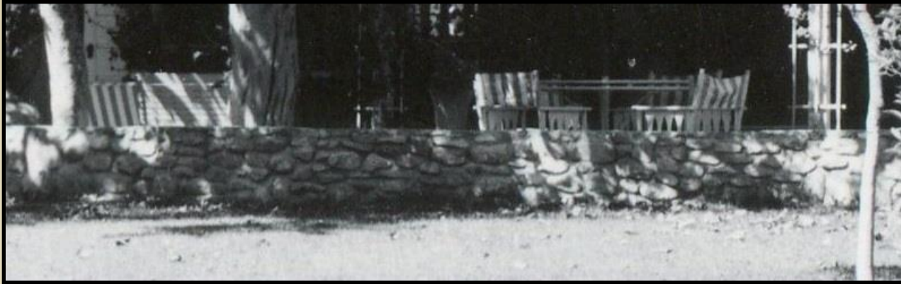
Retaining walls in front of the patio at the house
