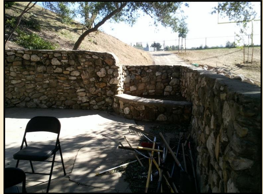
BBQ patio looking south
